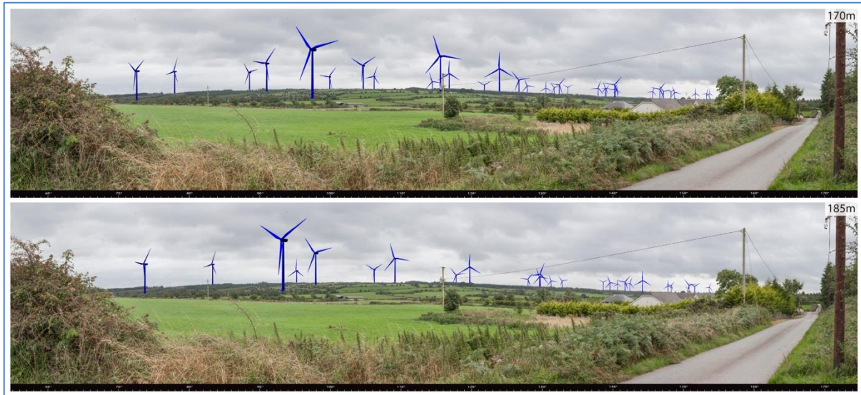
Figure 13-23: Early stage height versus density relationship study (33 no. 170m TH and 25 no. 185m TH) for Castlebanny turbines (looking SE from local road near Mountainview Golf Course) – superseded layout
